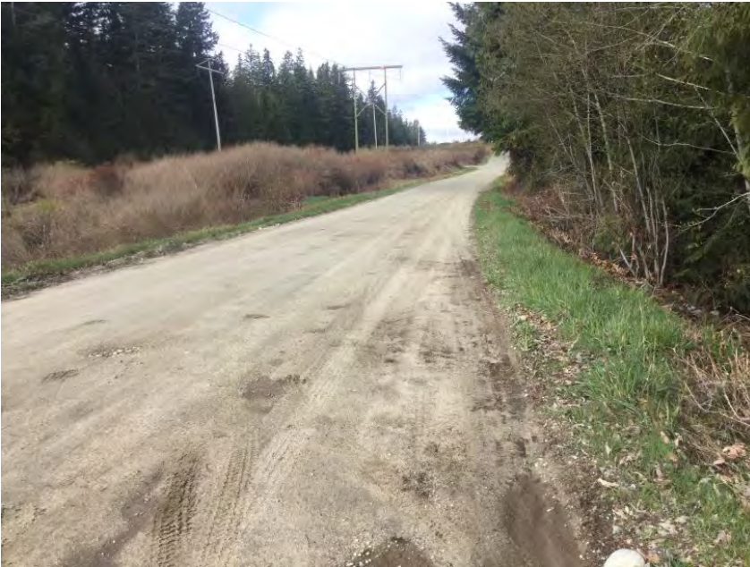
Approach from Left Bank when facing downstream
