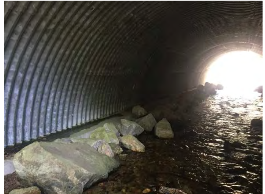
Left Bank Abutment when facing downstream
