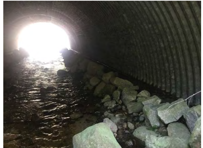
Right Bank Abutment when facing downstream
